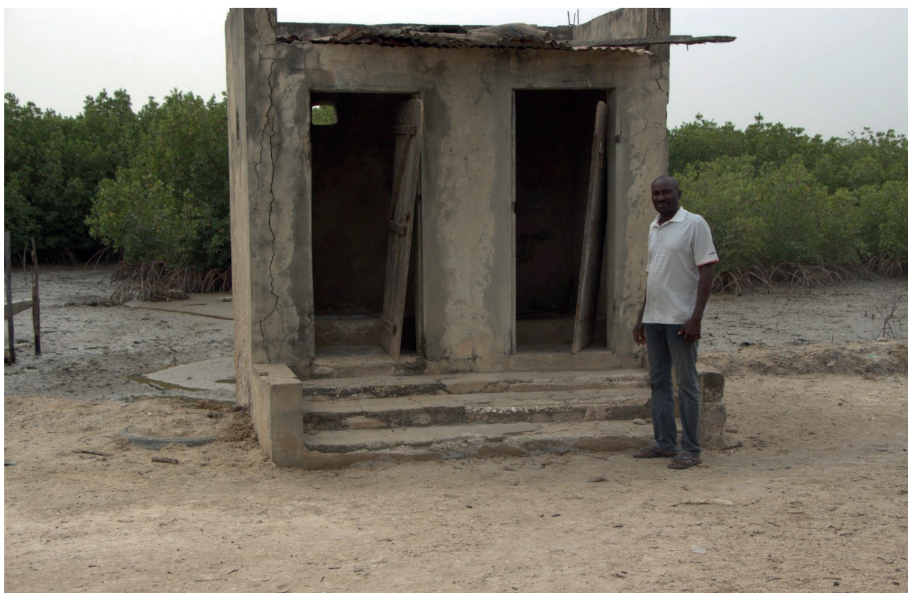
Community latrines on the islands of Lower Casamance © ISE-IPAR, 2024
